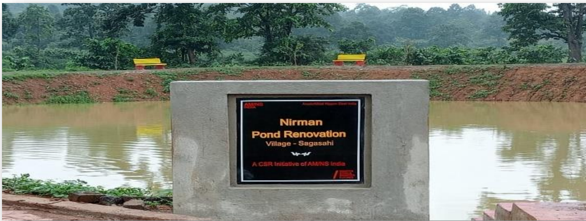
Pond renovation at Sagasahi
